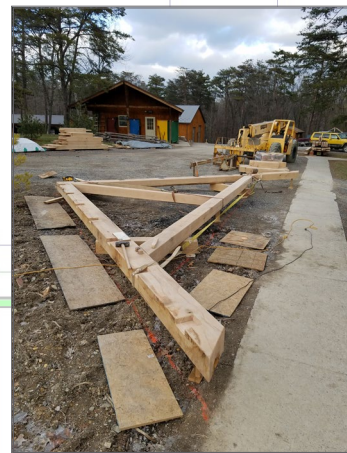
THE FIRST TRUSS IS ASSEMBLED
